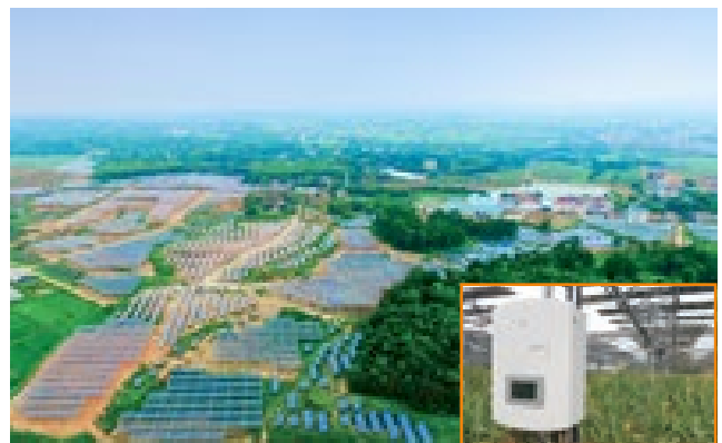
Quzhou Qinghu Agricultural-photovoltaic hybrid PV plant 20MW
