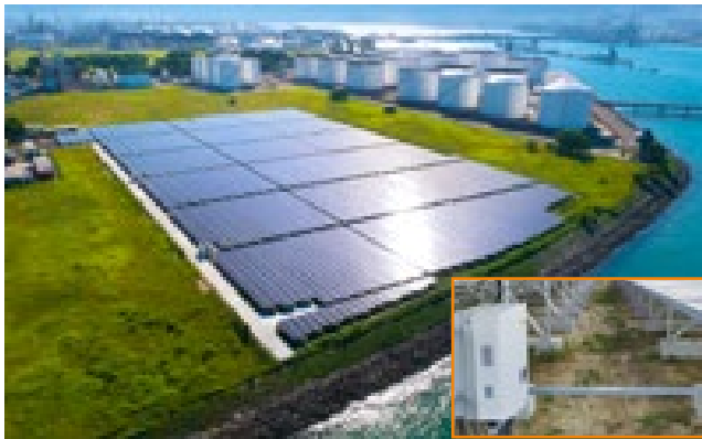
JTC Solar Farm, Singapore 5MW
