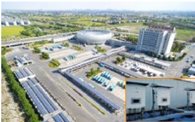
Zhejiang PINGHU Bus Station 472kW
