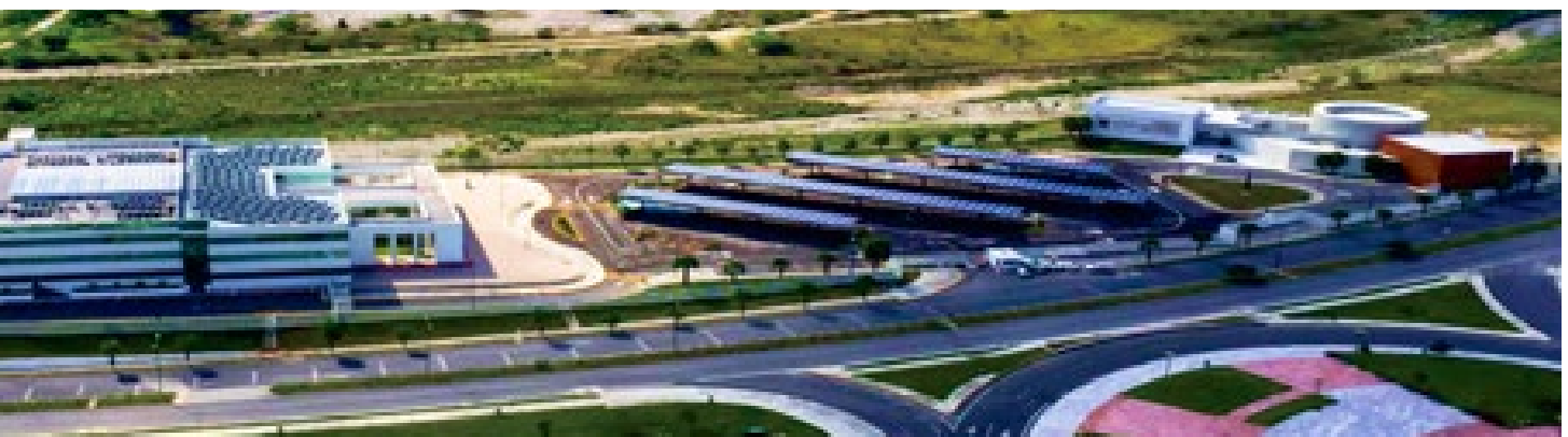
Mexico-Tamaulipas Carport, Mexico 5MW
